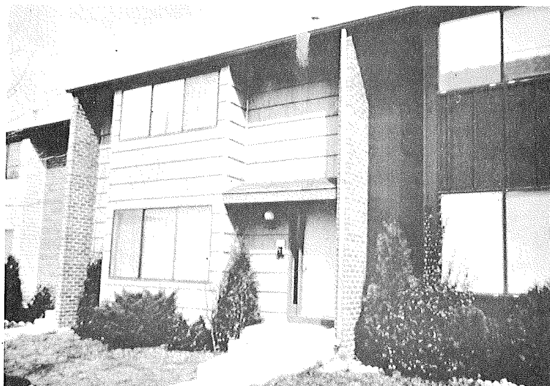
FRONT VIEW OF QUAD II TOWNHOUSE RENTED BY PRINCETON. MASONRY FIREWALLS PROJECT BEYOND THE STRUCTURE IN BRICK. CENTRAL PROJECTION (WITH WINDOWS OF LIVING ROOM AND MASTER BEDROOM) TERMINATES ONE FOOT ABOVE GROUND LEVEL (BEHIND BUSHES).
