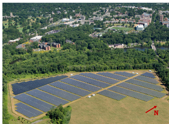
Figure A.1 Aerial view of the Princeton University photovoltaic field. The northern-most and western-most solar panels that appear darker are fixed-tilt panels; all of the others are tracking panels.
