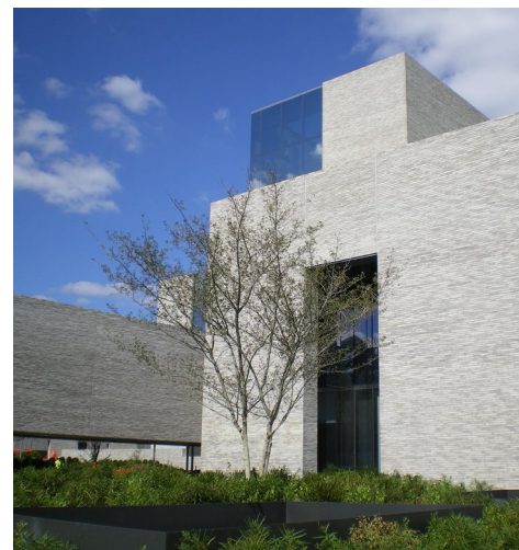
Andlinger Center, view from Olden Street.
