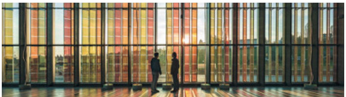
Figure 3.15: SwissTech Convention Center installation of dye-sensitized solar cells in a large glazed wall. The cells help prevent overheating in the afternoon while simultaneously generating electricity. Source: © FG+SG fotografie de architectura, http://www.detail-online.com/inspiration/report-the-cutting-edge-of-research-%E2%80%93-epfl%E2%80%99s-swisstech-convention-center-111842.html .
