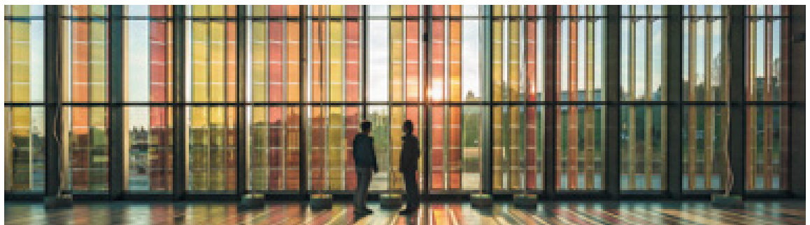
Figure 3.15: SwissTech Convention Center installation of dye-sensitized solar cells in a large glazed wall. The cells help prevent overheating in the afternoon while simultaneously generating electricity. Source: © FG+SG fotografie de architectura, http://www.archdaily.com/519434/epfl-quartier-nord-swisstech-convention-center-retail-and-student-housing-richter-dahl-rocha-and-associates/53a84e94c07a80c112000101-epfl-quartier-nord-swisstech-convention-center-retail-and-student-housing-richter-dahl-rocha-and-associates-photo .
