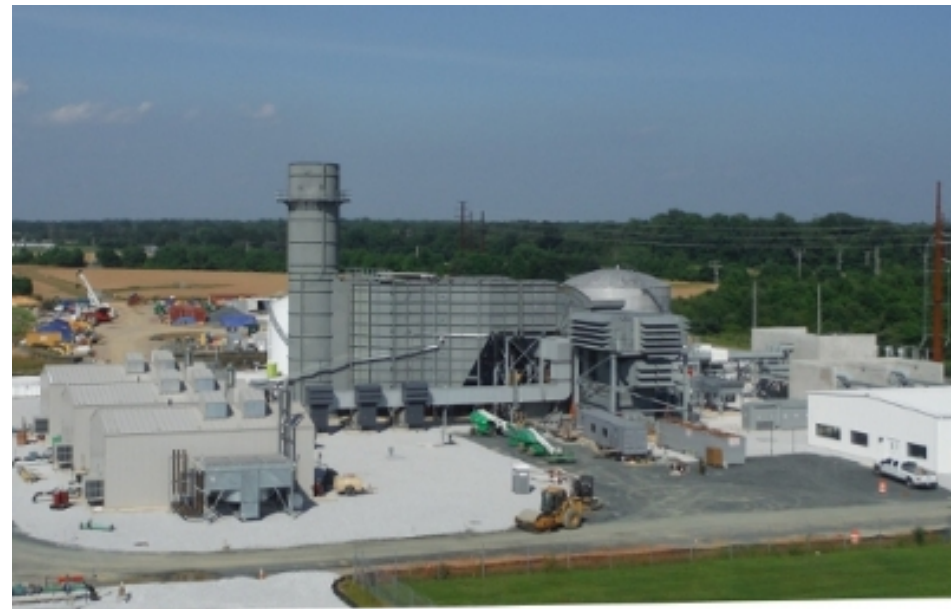
Natural Gas Plant
