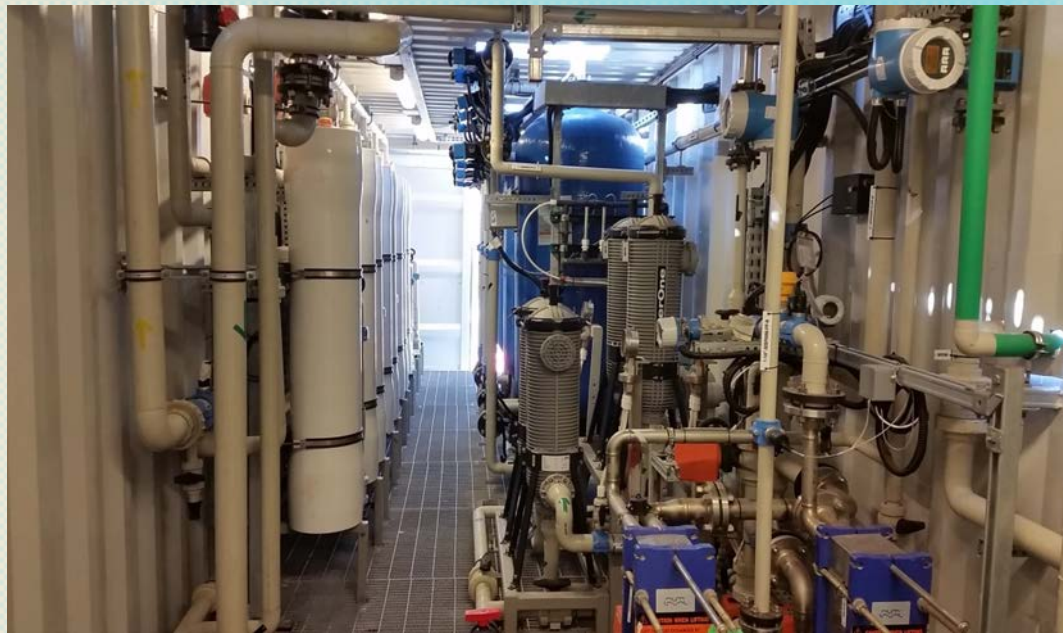
System in operation, producing WHO quality water at <1.0\text{kWh}/\text{m}^3 .
